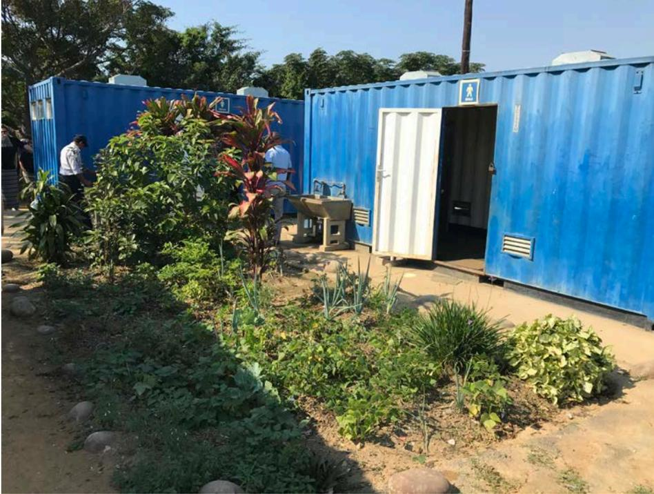
Figure 3. Container-based platforms called Community Ablution Blocks (CABs) provide sanitation and hygiene service to informal settlements in Durban, South Africa. The NEWgenerator will be coupled with CABs to provide onsite wastewater treatment and water recycling.
